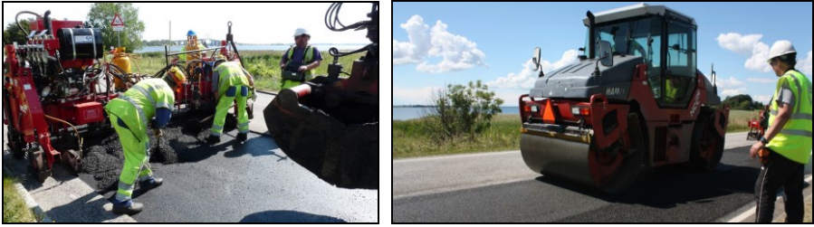
Figure 8: Construction of the first Danish full scale test track in Kalvehave (Kalvehave I): the fresh PERS mix in front of the gussasphalt paver was first spread manually (left hand side) and then compacted (right hand side)
